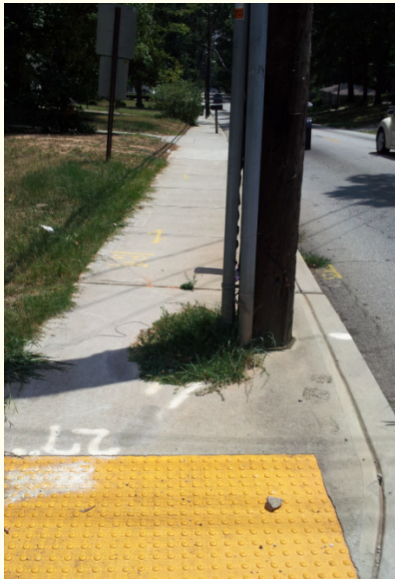
Obstructions within the pedestrian route
