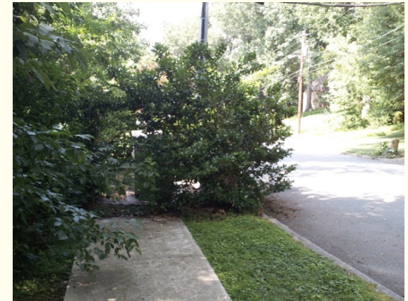
Insufficient vertical clearance
